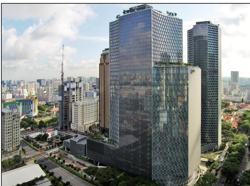
The Duo, Singapore, where both of its towers' walls are post-tensioned due to the unbalanced geometry of the structure.
