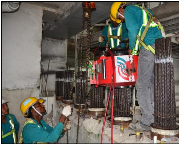
Stressing of vertical tendons in progress
