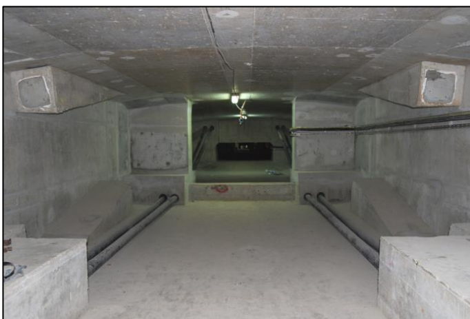
Completed external tendons
